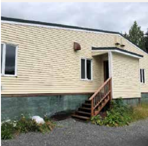
The Eyak Corporation Building on LeFevre Drive.
